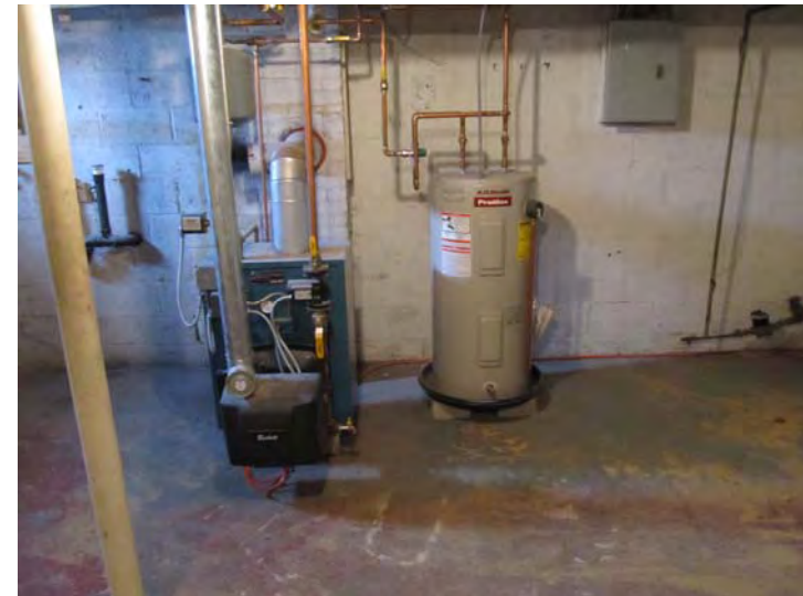
Newer unit level boiler for hydronic heat and indirect-fired domestic hot water tank – Newest replacement tanks are freestanding electric models
