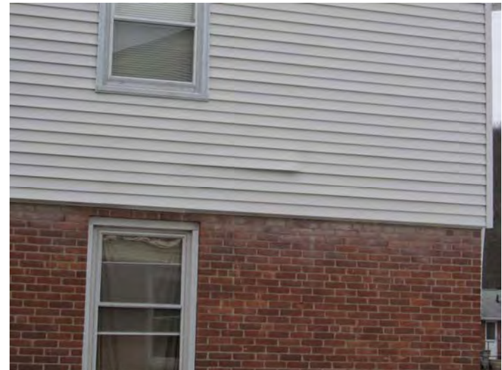
Isolated loose vinyl siding seams noted at various locations
