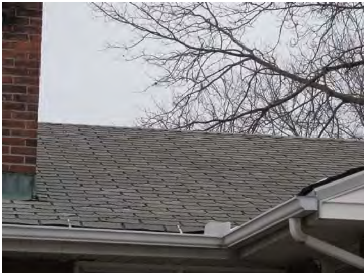
Older three-tab roof shingles exhibit age-related wear and deterioration
