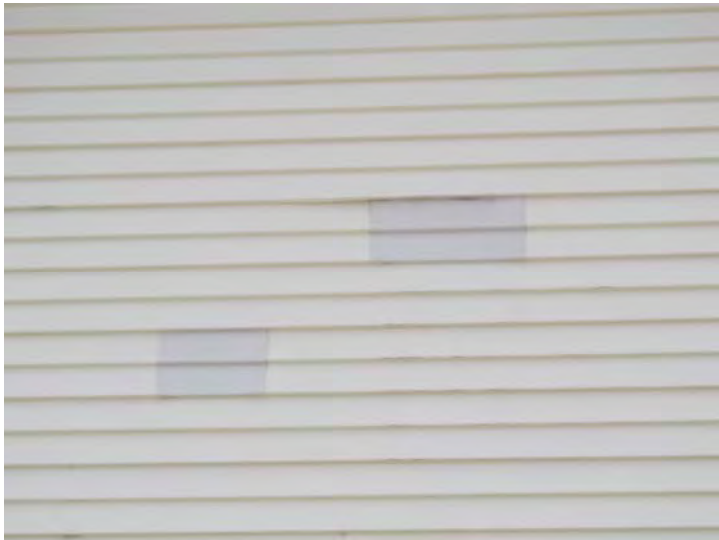
Past vinyl siding patch repairs also noted at various locations
